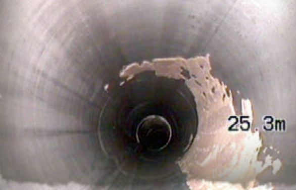
An in-line camera shows significant milk stone build-up 25.3mm into the line.
