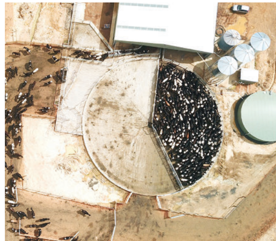
Rod and Jess Warren had the complete picture in mind when they mobilised their dairy build.
